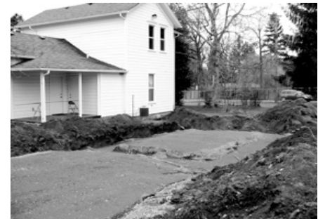
Heslin House, South Side & Future Garage
